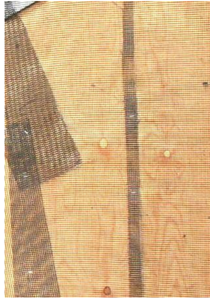
Fig.7. G-ES netting, overlapping pieces, nailed against wood board
