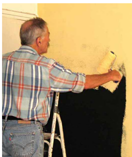
Fig. 11. Two layers of decorative paint are necessary for making the black invisible.
