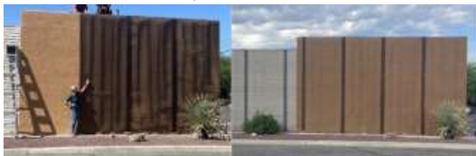
Safe Tech Tucson volunteers attaching metal mesh screening to the external wall of a school room during the demonstration cell tower radiation shielding in November 2023.
